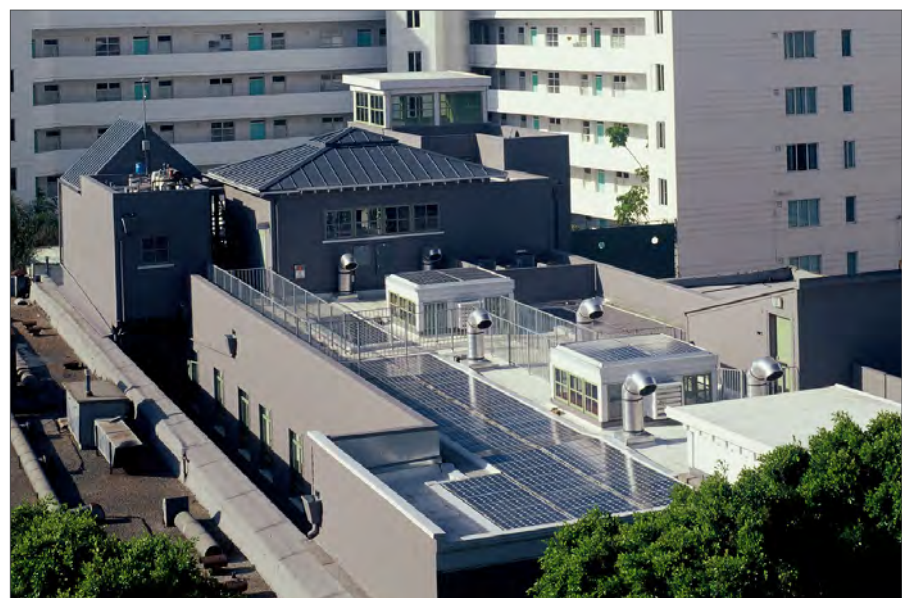
An office building utilizes rooftop solar panels and natural light and ventilation from rooftop light monitors.
