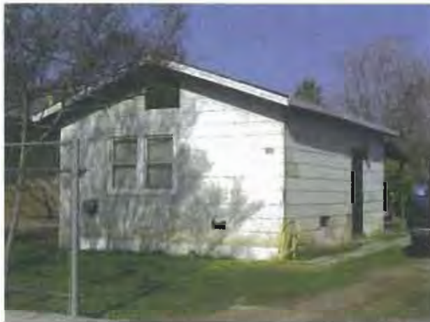
PHOTO 43 Dilapidated residence with asbestos shingle siding. APN 464 142 19 1613 AY
