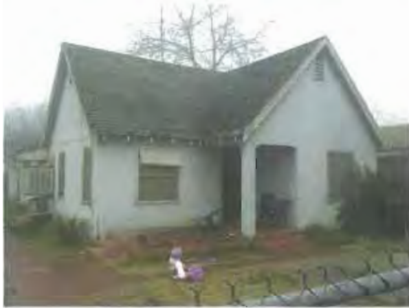
PHOTO 31 Dilapidated residence on Atchison Avenue. APN 478 253 12 1504 AY
