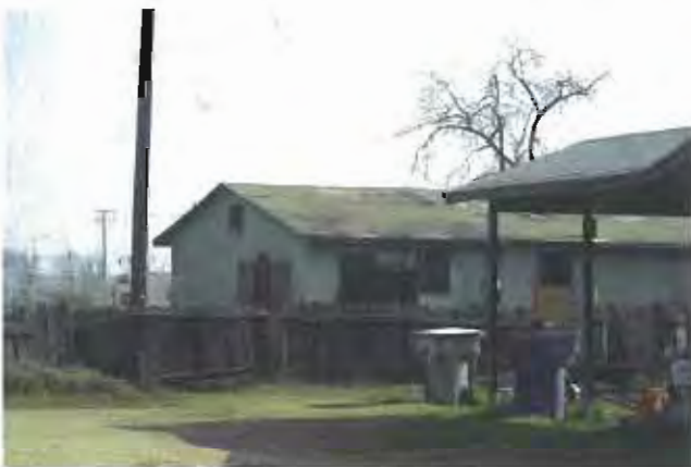
PHOTO 15 Dilapidated residence on Poppy Avenue. APN 328 150 17 08732 KG
