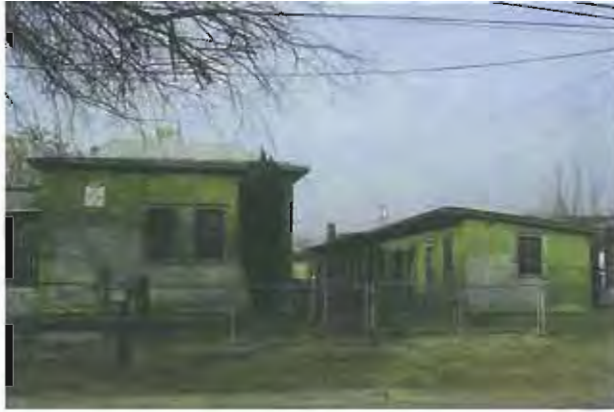
PHOTO 9 Dilapidated residences on Belgravia Avenue. APN 477 132 02 08654 KG
