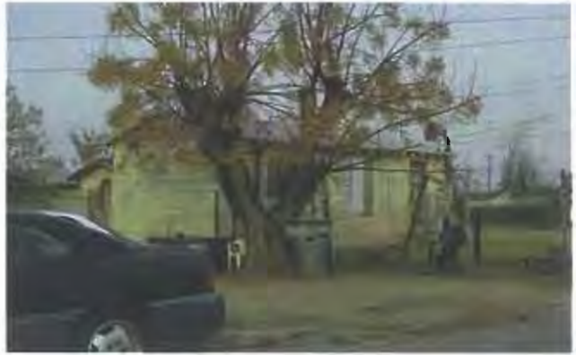
PHOTO 2 Dilapidated residence on Eunice Ave. APN 477 113 05 08661 KG
