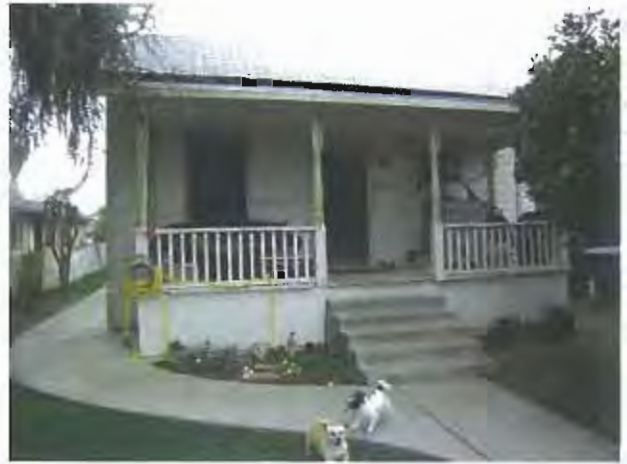
PHOTO 34 Dilapidated residence APN 467 172 13 1527 AY
