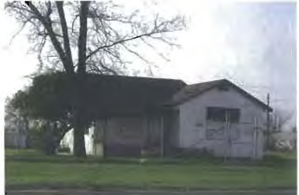
PHOTO 74 Dilapidated, boarded up residence on B Street. APN 458 212 36 08686 KG
