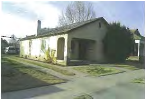
PHOTO 23 Deteriorated residence on California Ave. APN 478 201 12 1464 AY
