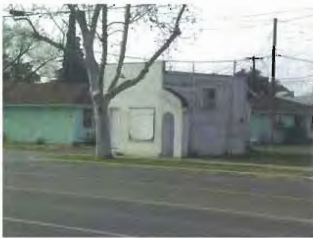
PHOTO 67 Dilapidated, obsolete commercial building on Samson Ave. APN 467 251 08 1545 AY
