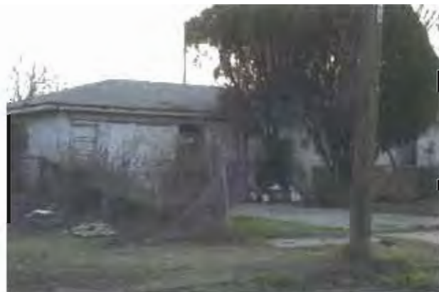
PHOTO 18 Dilapidated residence on Florence Avenue. APN 328 252 12 08742 KG
