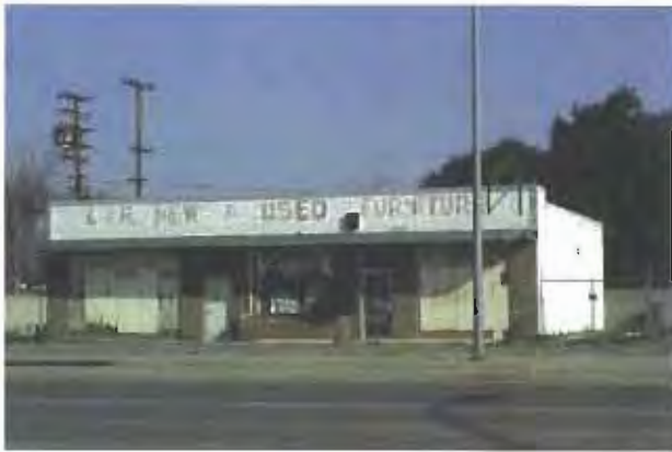
PHOTO 65 Dilapidated commercial building. APN 479 211 10 8746 KG
