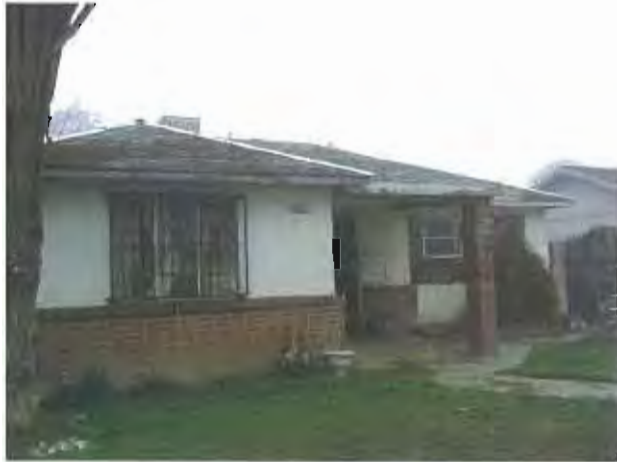
PHOTO 49 Dilapidated residence on Ivy Avenue. APN 478 252 17 0031 JL
