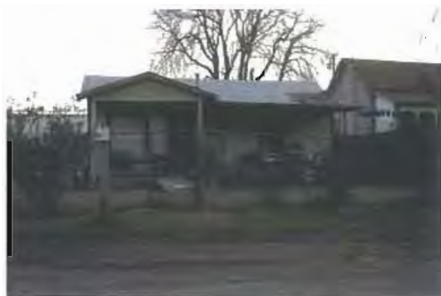
PHOTO 17 Dilapidated residence on Belgravia Avenue. APN 328 252 15 08741 KG
