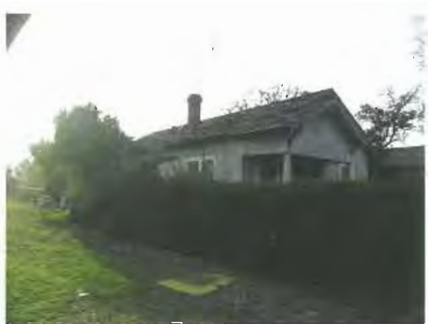
PHOTO 40 Dilapidated residence on C Street. APN 465 174 06 1579 AY
