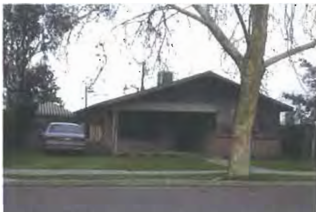
PHOTO 19 Deteriorated residence on C Street. APN 465 125 15 08694 KG
