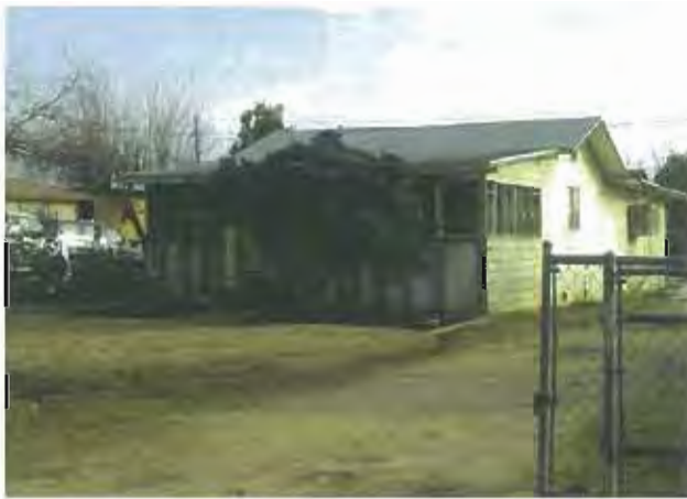
PHOTO 11 Dilapidated residence APN 477 134 04 08614 KM
