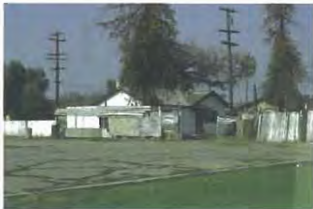
PHOTO 13 Dilapidated residence on San Joaquin Street. APN 458 220 26 08710 KG
