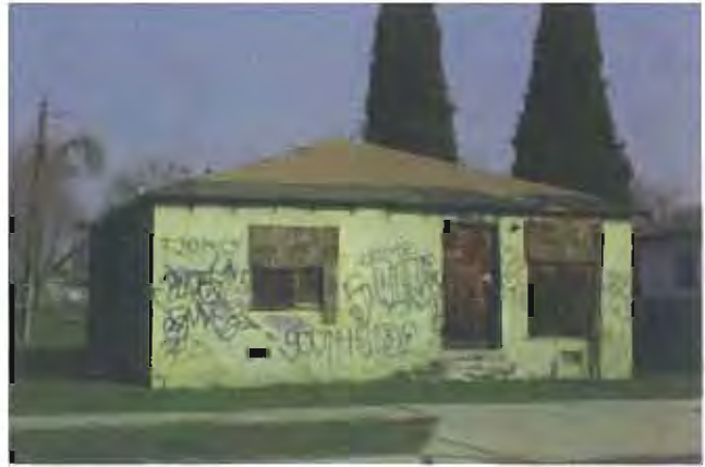
PHOTO 70 Dilapidated residence on Oleander Avenue. APN 464 113 13 08704 KG
