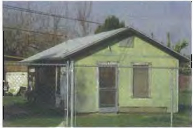
PHOTO 10 Dilapidated residence with asbestos shingle siding and no foundation. APN 477 134 17 8650 KG
