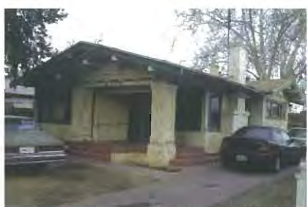
PHOTO 24 Deteriorated residence on Banneker Avenue. APN 478 144 21 1474 AY
