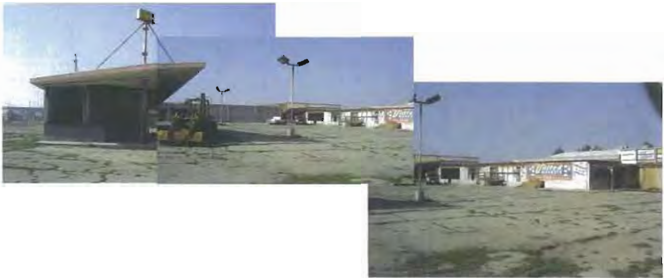
PHOTOS 63 and 64 Dilapidated and obsolete commercial buildings. APN 328 150 10 8727 through 8729 KG
