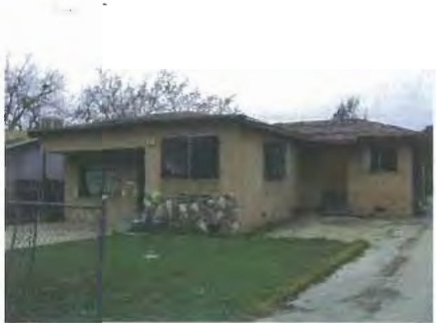
PHOTO 50 Dilapidated residence. APN 478 065 09 0040 JL
