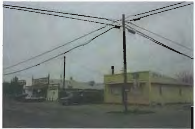
PHOTO 78 Deteriorated and obsolete commercial buildings on Whites- bridge Avenue.. APN 329 161 46 8670 KG
