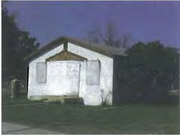
PHOTO 89 Dilapidated, boarded up residence on Chandler Ave. APN 464 192 14 1615 AY
