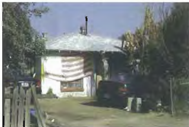
PHOTO 14 Dilapidated residence APN 328 150 25 08724 KG
