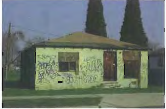
PHOTO 70 Dilapidated residence on Oleander Avenue. APN 464 113 13 08704 KG
