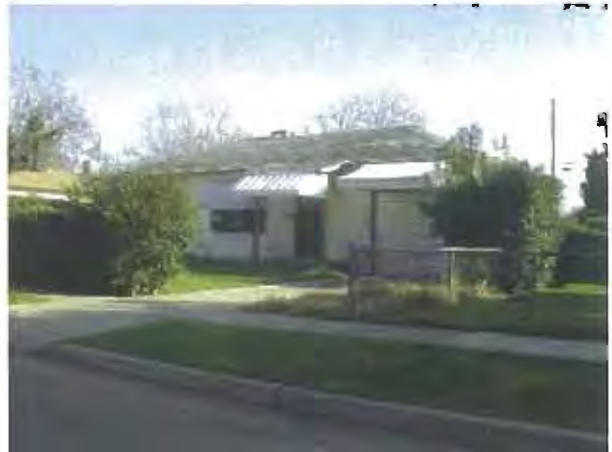
PHOTO 8 Deteriorated residence APN 479 174 14 8638 KM
