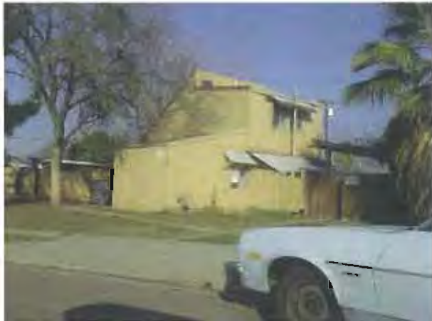
PHOTO 7 Dilapidate residence on B Street APN 328 172 40 8631 KM
