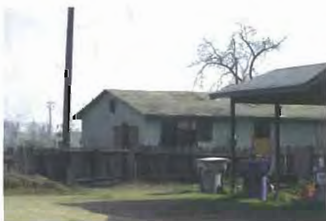
PHOTO 15 Dilapidated residence on Poppy Avenue. APN 328 150 17 08732 KG
