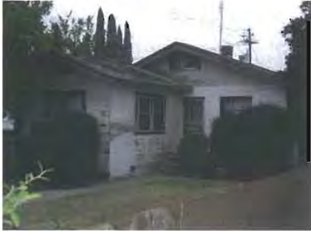
PHOTO 33 Dilapidated residence on Thorne Avenue. APN 467 232 11 1518 AY
