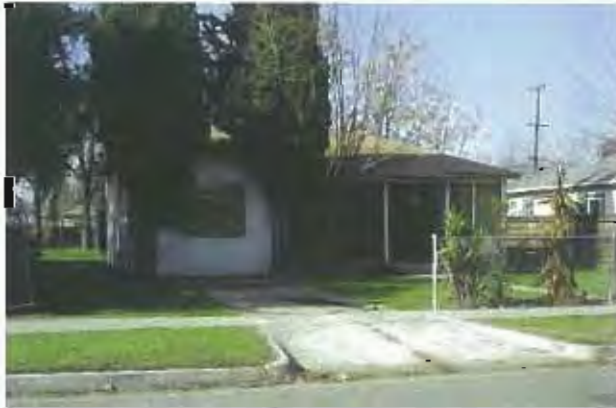
PHOTO 75 Dilapidated residence on Teilman Avenue. APN 479 211 10 08744 KG
