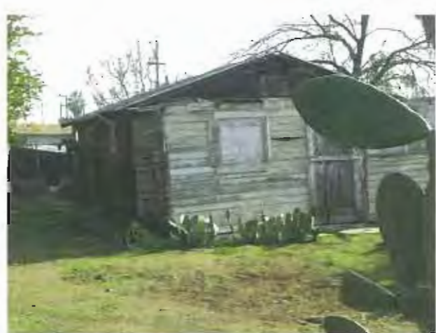
PHOTO 88 Dilapidated residence on Holly Avenue. APN 465 232 13 1563 AY
