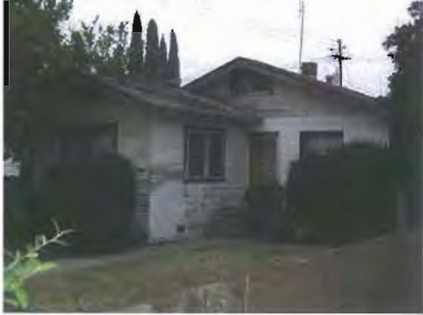
PHOTO 33 Dilapidated residence on Thorne Avenue. APN 467 232 11 1518 AY
