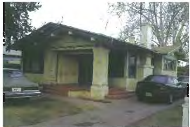
PHOTO 24 Deteriorated residence on Banneker Avenue. APN 478 144 21 1474 AY
