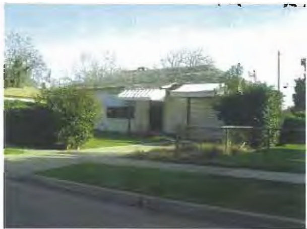
PHOTO 8 Deteriorated residence APN 479 174 14 8638 KM
