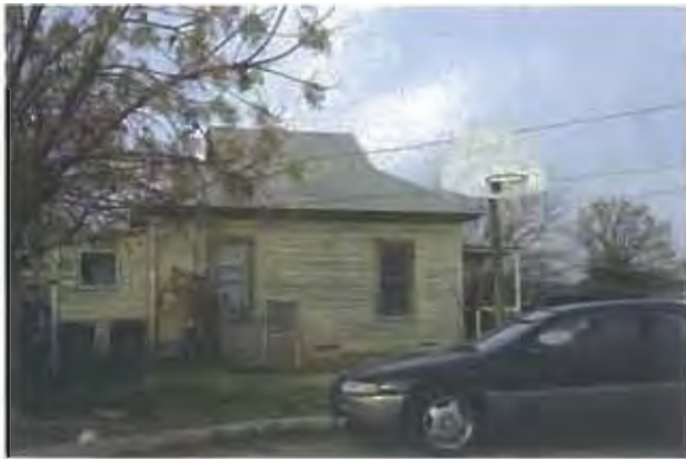
PHOTO 1 Dilapidated residence on Ivy Avenue. APN 477 113 06 08660 KG
