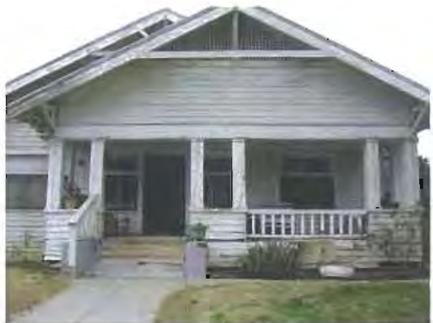
PHOTO 52 Dilapidated residence with a foundation in need of repair on Tupman Avenue. APN 467 166 13 0046 JL
