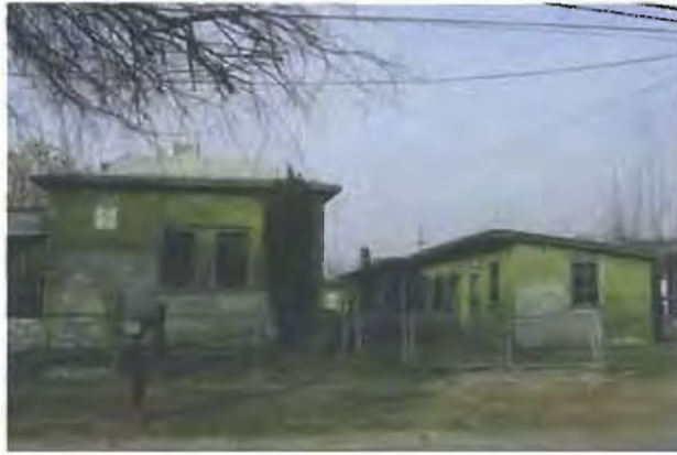
PHOTO 9 Dilapidated residences on Belgravia Avenue. APN 477 132 02 08654 KG
