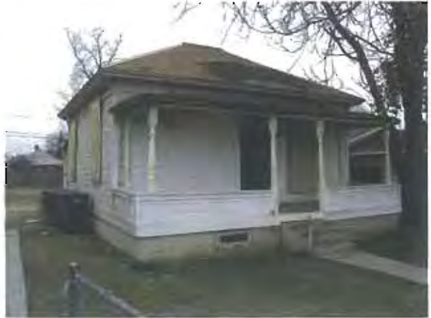
PHOTO 86 Deteriorated residence with foundation and roof in need of repair on Elm Avenue. APN 467 214 07 1541 AY
