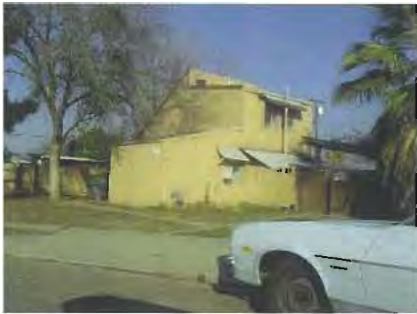
PHOTO 7 Dilapidate residence on B Street APN 328 172 40 8631 KM
