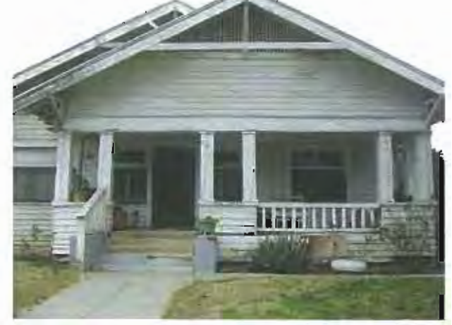
PHOTO 52 Dilapidated residence with a foundation in need of repair on Tupman Avenue. APN 467 166 13 0046 JL
