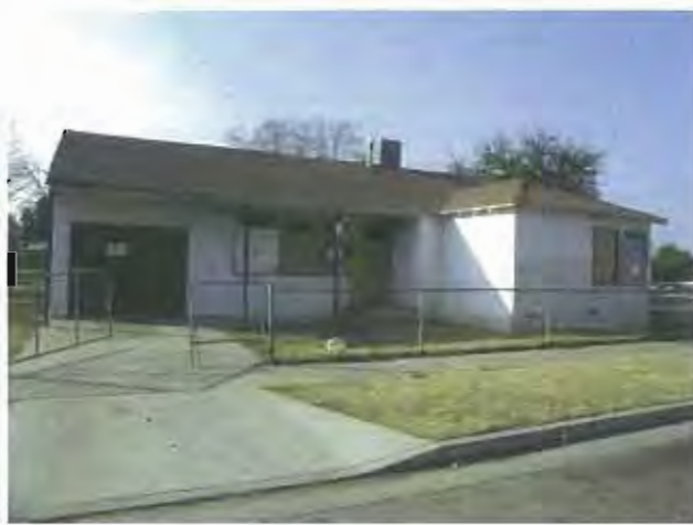
PHOTO 87 Dilapidated, boarded up residence on Fruit Avenue. APN 465 191 05 1571 AY
