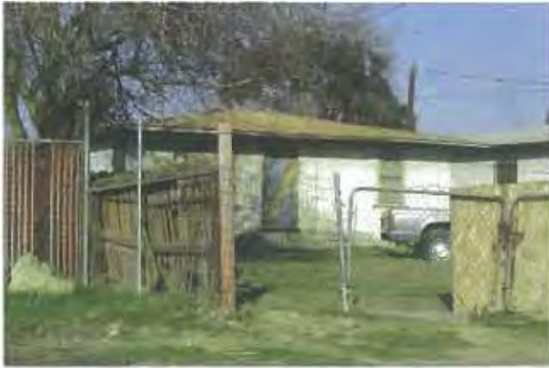
PHOTO 21 Deteriorated residence on Valencia Avenue. APN 329 161 22 08748 KG
