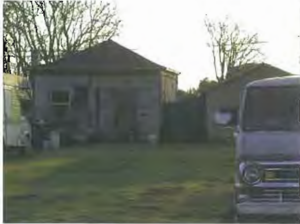
PHOTO 41 Dilapidated residence on North Avenue. APN 467 155 04 1585 AY
