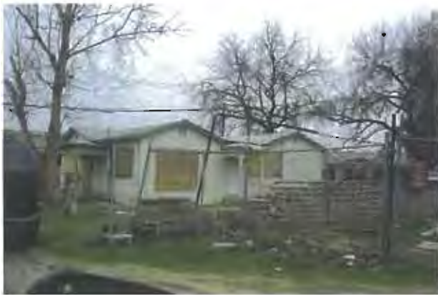
PHOTOS 71 and 72 Dilapidated, abandoned residence with holes in the foundation and adjacent failing retaining wall on Holly Avenue. A portion of the building has been demolished. Dilapidated structures are visible behind the building. APN 458 230 01 08682, 08684 KG
