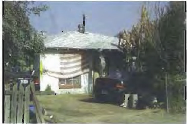
PHOTO 14 Dilapidated residence APN 328 150 25 08724 KG
