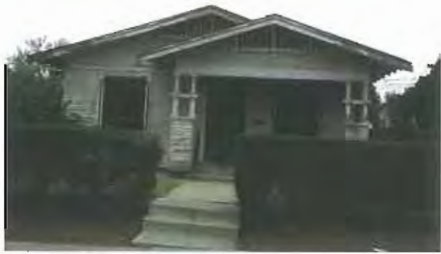
PHOTO 37 Dilapidated residence on Elm Avenue. APN 467 192 10 1543 AY
