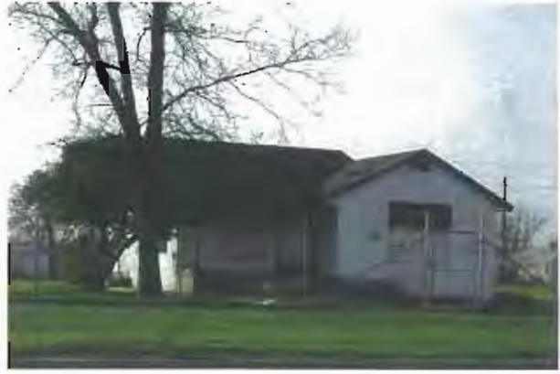
PHOTO 74 Dilapidated, boarded up residence on B Street. APN 458 212 36 08686 KG
