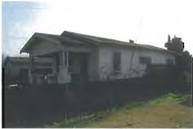
PHOTO 45 Dilapidated residence on Almy Ave. APN 465 216 04 1566 AY
