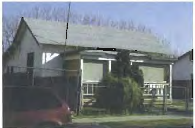
PHOTO 22 Dilapidated residence with asbestos shingle siding. APN 478 134 15 08757 KG
