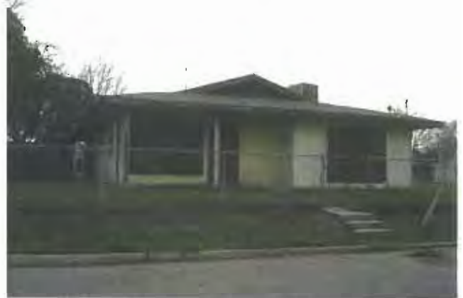
PHOTO 16 Deteriorated residence on Santa Clara Street. APN 477 114 06 08665 KG
