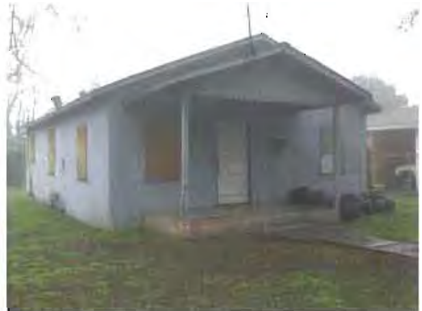
PHOTO 76 Dilapidated residence on Atchison Street. APN 478 252 08 1502 AY
