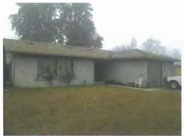
PHOTO 32 Dilapidated residence on Elm Avenue. APN 478 311 23 1505 AY
