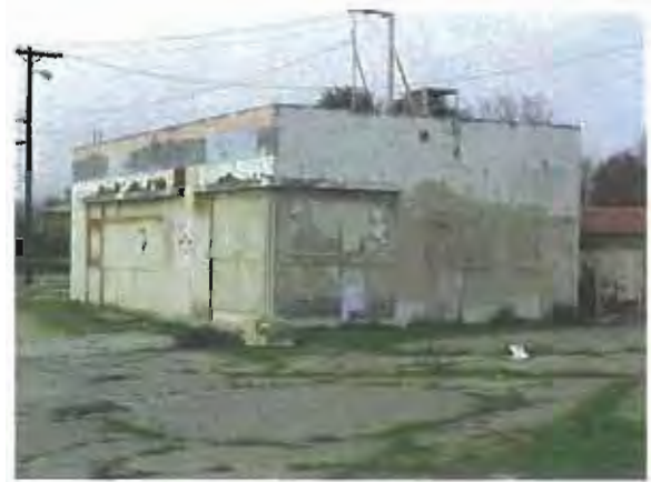
PHOTO 66 Dilapidated, abandoned commercial building on North Avenue. APN 467 246 01 1544 AY
