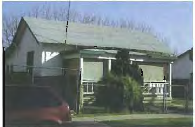
PHOTO 22 Dilapidated residence with asbestos shingle siding. APN 478 134 15 08757 KG
