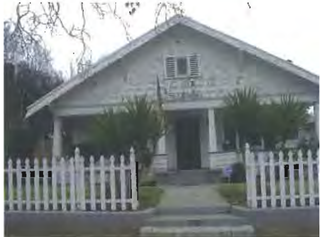
PHOTO 12 Dilapidated residence with failing foundation. APN 467 166 14 08625 KM
