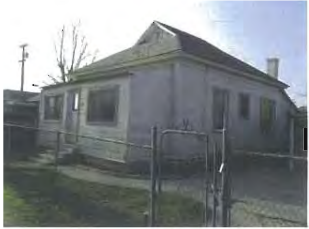
PHOTO 38 Dilapidated residence on Tupman Ave. APN 465 172 08 1573 AY
