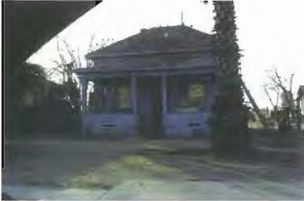
PHOTO 73 Dilapidate residence on Woodward Avenue. APN 328 150 36 08739 KG
