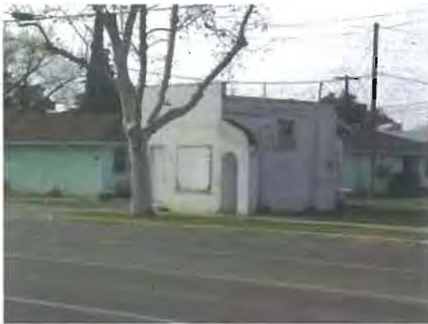
PHOTO 67 Dilapidated, obsolete commercial building on Samson Ave. APN 467 251 08 1545 AY
