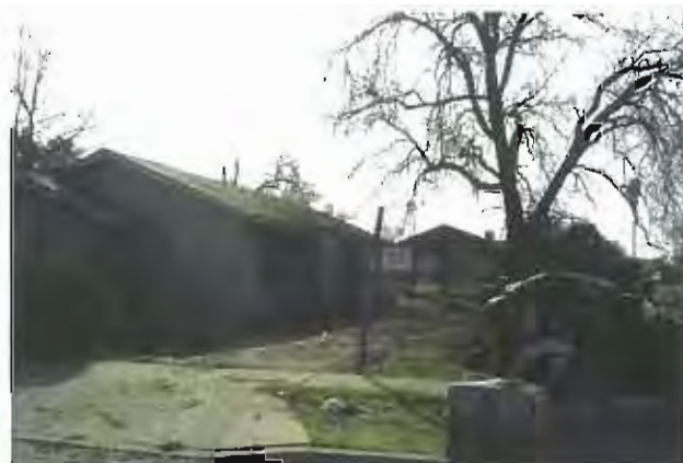
PHOTO 28 Dilapidated residence on Lotus Avenue. APN 464 121 33 08707 KG
