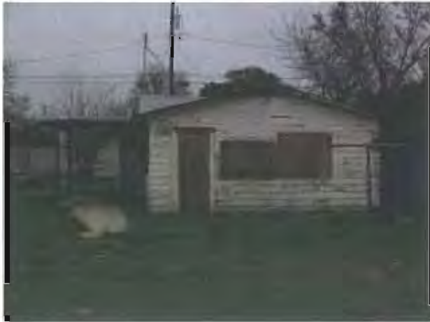
PHOTO 85 Dilapidated, boarded-up residence. APN 467 184 14 1521 AY
