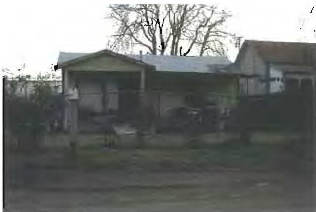
PHOTO 17 Dilapidated residence on Belgravia Avenue. APN 328 252 15 08741 KG
