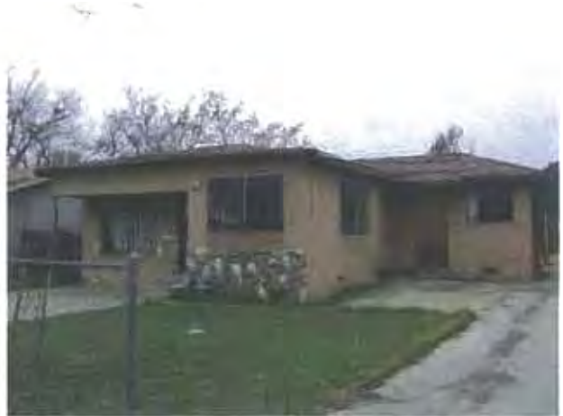
PHOTO 50 Dilapidated residence. APN 478 065 09 0040 JL
