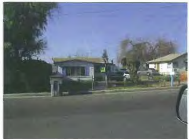
PHOTO 44 Dilapidated residence APN 464 080 09 1614 AY
