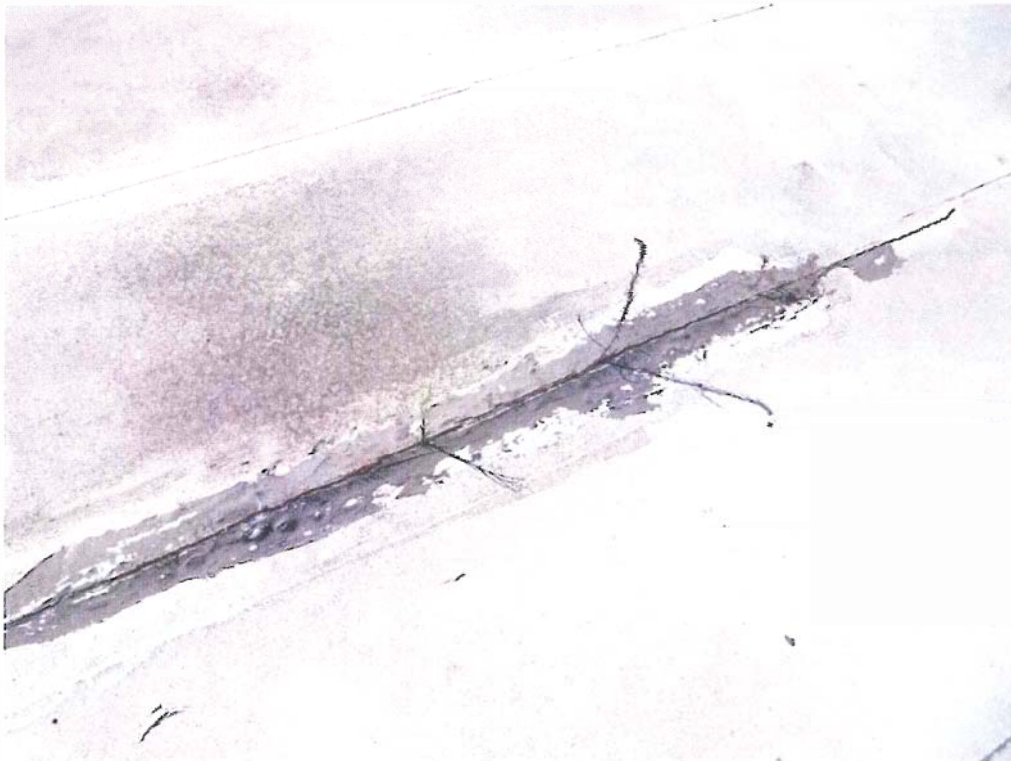
Photograph Number 6 Failed Split Repair in Field of Roof
