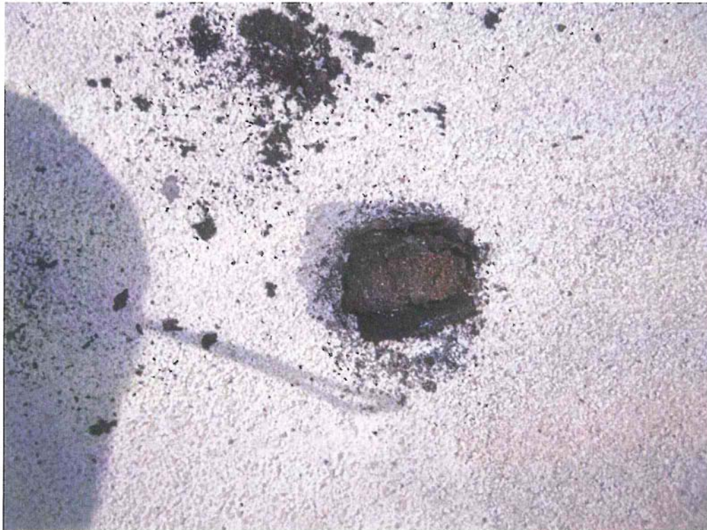
Photograph Number 16 Close-Up of Roof Core
