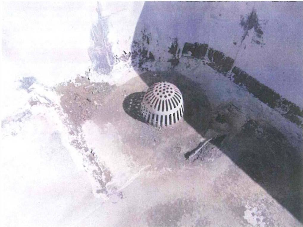
Photograph Number 4 Typical Roof Drain
