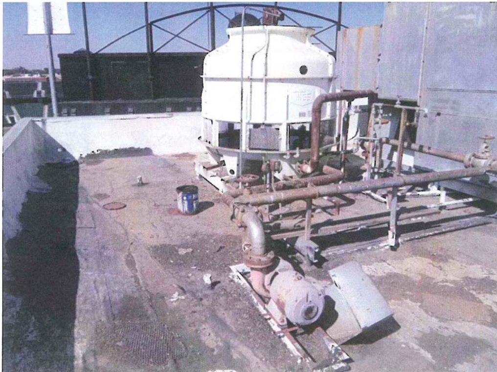
Photograph Number 14 Field Repairs at Mechanical Area
