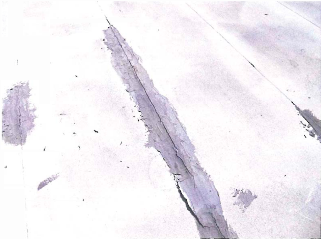
Photograph Number 7 Failed Split Repair
